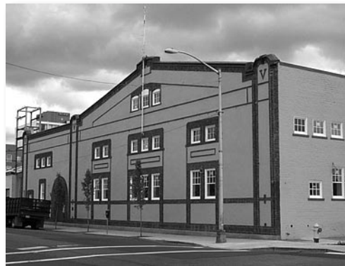
American Legion Building renovated in 2003. Olympia Heritage Commission photo.
