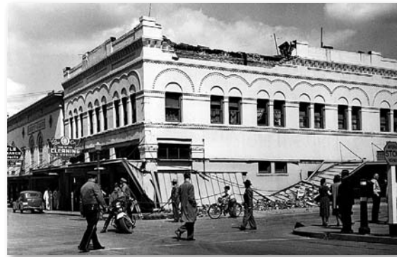
Damage after the 1949 earthquake, corner of Legion Way and Washington St. The Liberty Theatre can be seen at the left, where the Washington Center for the Performing Arts stands today. The damaged building in the center of the photo is the historic Reed Block—current location of Drees. Olympia Heritage Commission Collection.
