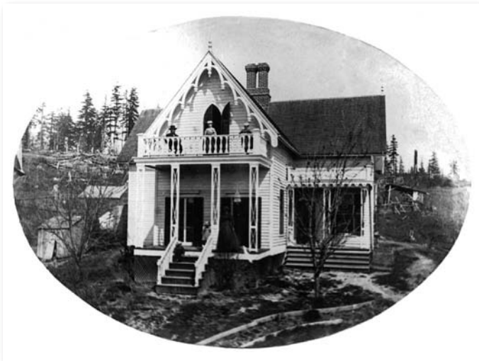
The Bigelow House as it appeared during the 1860s. The Carpenter Gothic style borrowed elements from medieval church architecture and reinterpreted them in wooden construction: a steeply pitched roof, gothic (pointed) arches, decorative millwork that suggested the carved stone of old cathedrals. It was a style that peaked in popularity back east at about the time early pioneer settlers were moving west. The Bigelow House Museum Collection.
