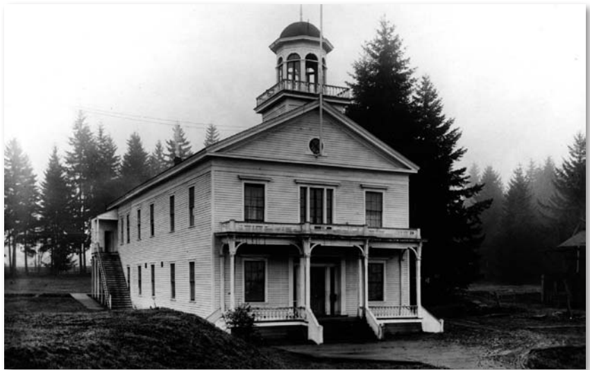
Washington's first capitol stood at the top of the hill behind town on the site of the present Capitol Campus. A rear addition, just visible in this photograph, was built to accommodate the Constitutional Convention in 1889. Asahel Curtis photo (negative #1403), Special Collections Division, University of Washington Libraries.
