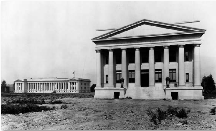
The first two buildings of the Capitol Group, the 1917 Temple of Justice, left, and the 1921 Insurance Building. Jeffers Photograph, J. Johnston papers, Manuscripts and University Archives, University of Washington Libraries. NR, SR
