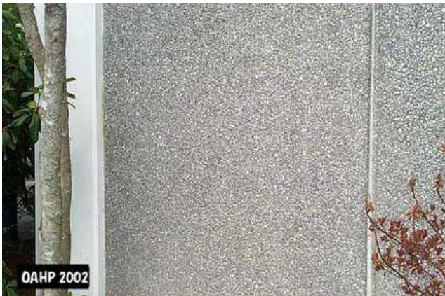
Marblecrete exterior finish.
