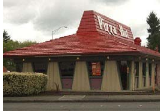
A Pizza Hut in neighboring Tumwater (c. 1970). Photo courtesy of the Department of Archaeology and Historic Preservation
