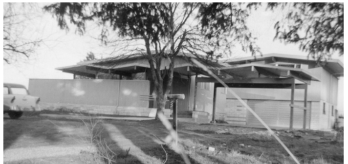
This house features a sawtooth roof on a covered garage. Photo courtesy of the Southwest Regional Branch of the Washington State Archives.
