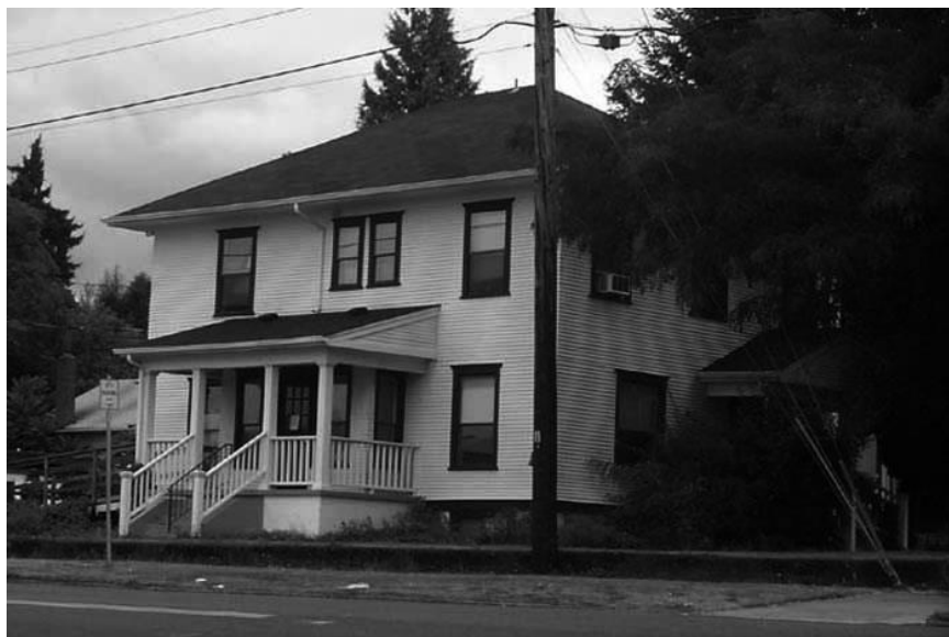
View of Front Facade taken 6/1/1901 Photography Neg. No. (Roll No./Frame No.): 3-2a Comments:
