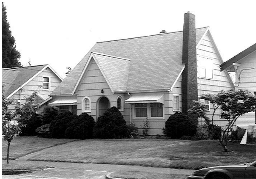
View of West Facade taken 7/13/1998 Photography Neg. No. (Roll No./Frame No.): 2 Comments:
