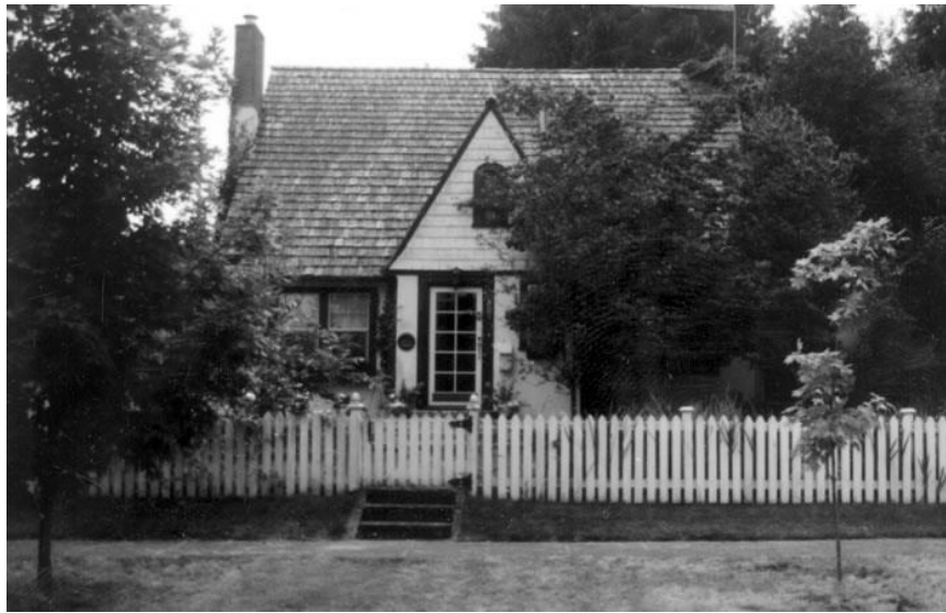
View of North Facade taken 7/1/1997 Photography Neg. No. (Roll No./Frame No.): 41-32A Comments:
