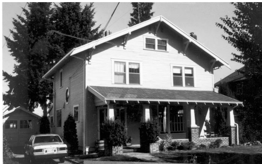
View of South Facade taken 7/1/1997 Photography Neg. No. (Roll No./Frame No.): 41-31 Comments:
