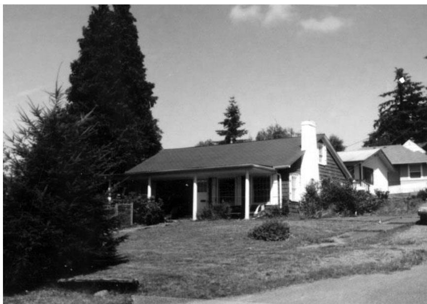
View of Southwest Facade taken 7/1/1997 Photography Neg. No. (Roll No./Frame No.): 42-32 Comments:
