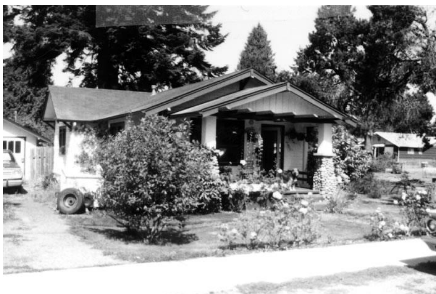
View of South Facade taken 8/1/1997 Photography Neg. No. (Roll No./Frame No.): 44-7 Comments:
