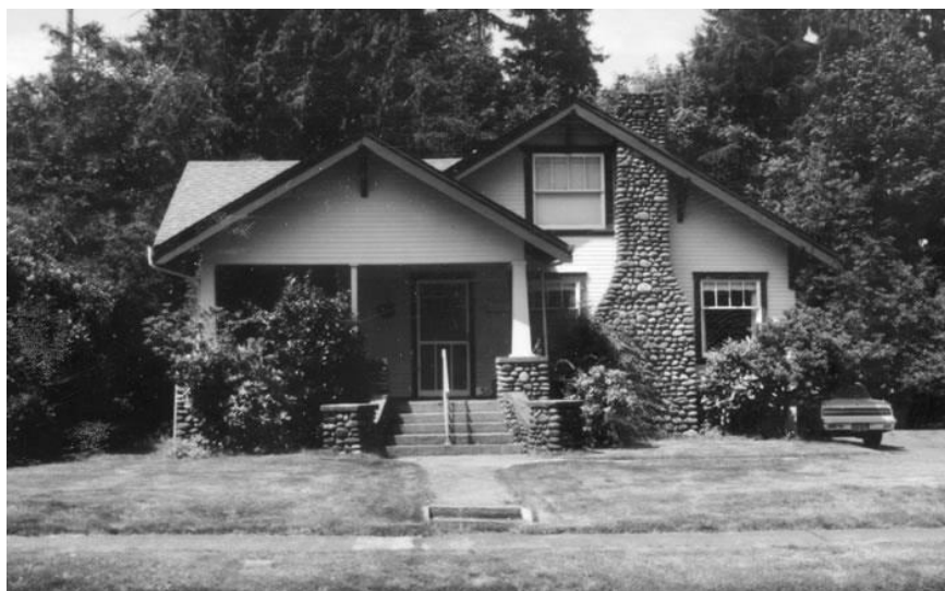
View of South facade taken 7/1/1997 Photography Neg. No. (Roll No./Frame No.): 42-20A Comments:
