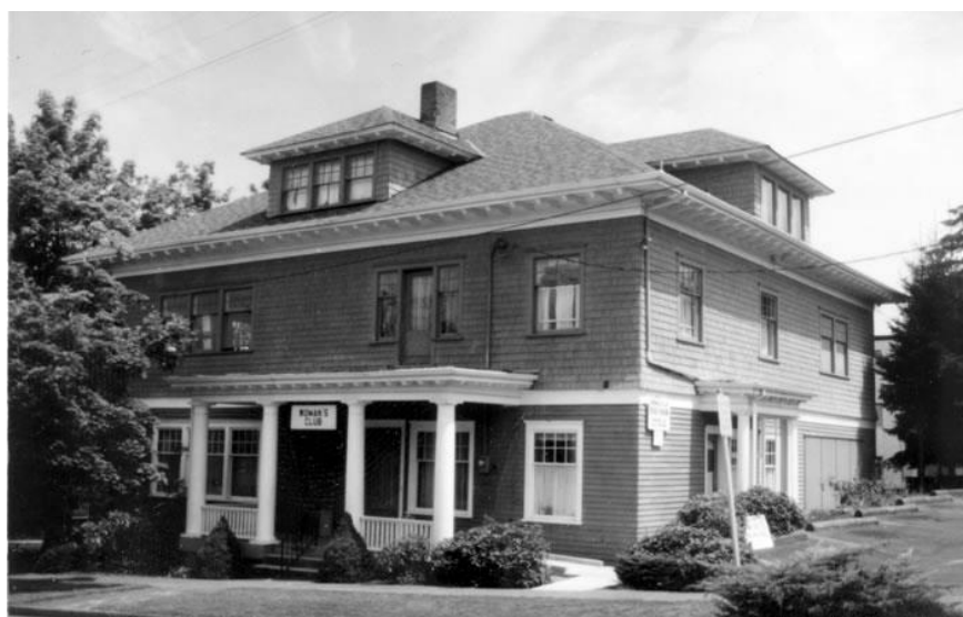
View of Southwest Facade taken 7/1/1997 Photography Neg. No. (Roll No./Frame No.): 41-15A Comments:
