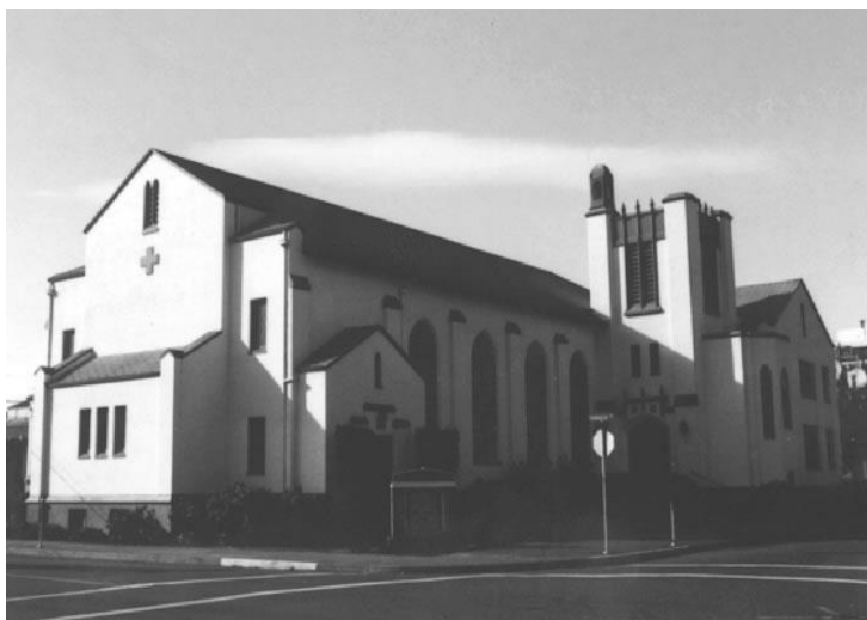
View of NE corner taken 10/17/1985 Photography Neg. No. (Roll No./Frame No.): 27-10A Comments:
