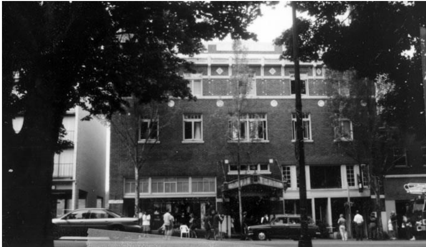
View of East Facade taken 10/16/1985 Photography Neg. No. (Roll No./Frame No.): 26-34A Comments:
