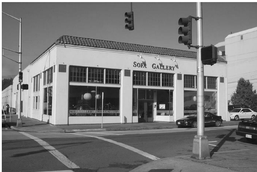
View of SE corner taken 10/16/1985 Photography Neg. No. (Roll No./Frame No.): 26-31A Comments:
