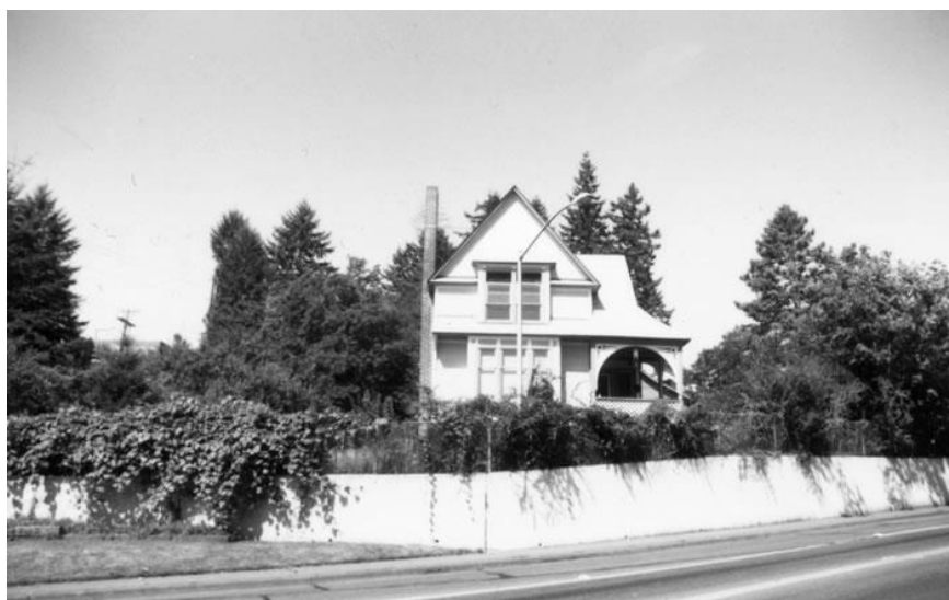
View of East Facade taken 9/1/1997 Photography Neg. No. (Roll No./Frame No.): 43-24 Comments:
