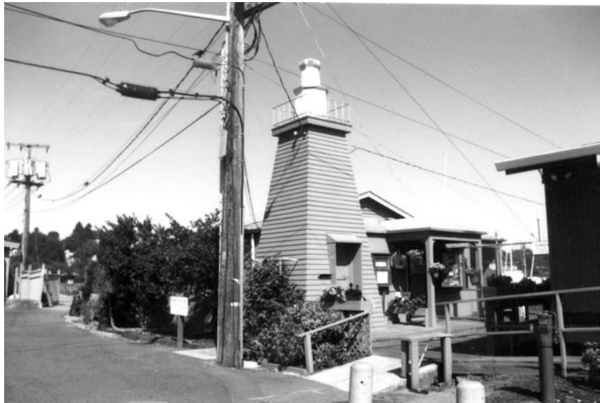
View of South Facade taken 9/1/1997 Photography Neg. No. (Roll No./Frame No.): 43-4 Comments:
