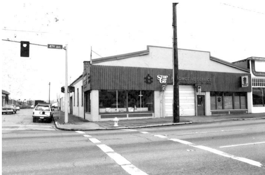
View of South facade taken 4/20/1990 Photography Neg. No. (Roll No./Frame No.): 39-17 Comments:
