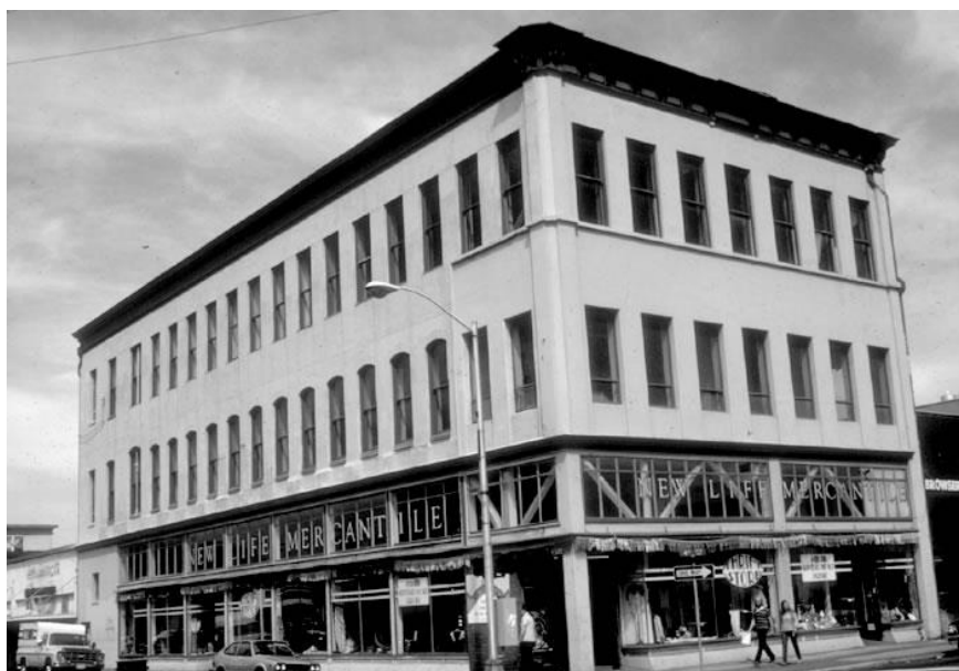
View of Southeast Corner taken 7/6/1989 Photography Neg. No. (Roll No./Frame No.): 38-1 Comments:
