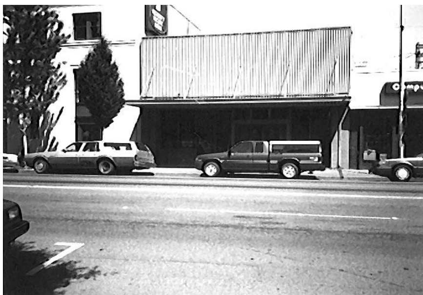
View of West Front Facade taken 6/5/1989 Photography Neg. No. (Roll No./Frame No.): 30-24A Comments:
