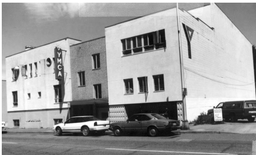
View of SW corner taken 7/6/1989 Photography Neg. No. (Roll No./Frame No.): 38-17 Comments:
