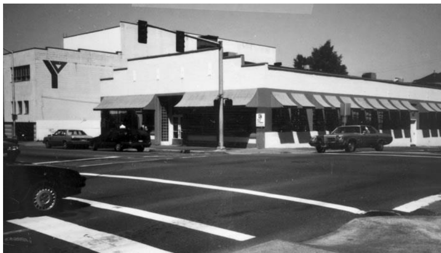
View of SW Corner taken 6/1/1989 Photography Neg. No. (Roll No./Frame No.): 37-20 Comments:
