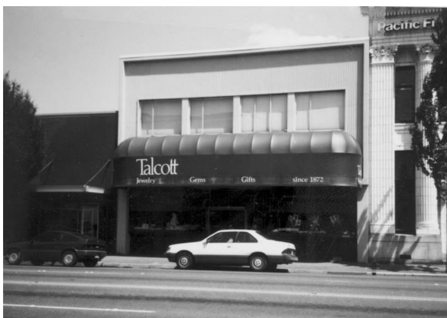
View of West (front) facade taken 5/31/1989 Photography Neg. No. (Roll No./Frame No.): 29-19 Comments:
