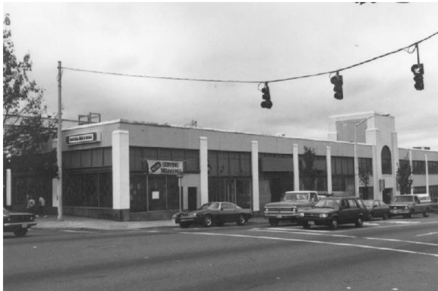
View of NE corner (shown); SE corner taken 10/17/1985 Photography Neg. No. (Roll No./Frame No.): 28-5.6 Comments:
