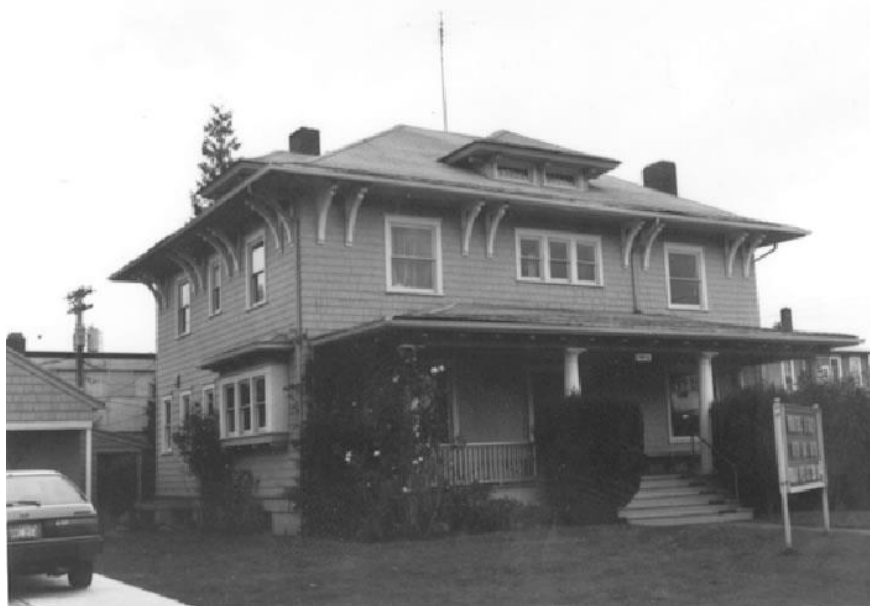
View of SW corner taken 10/17/1985 Photography Neg. No. (Roll No./Frame No.): 27-34A Comments:
