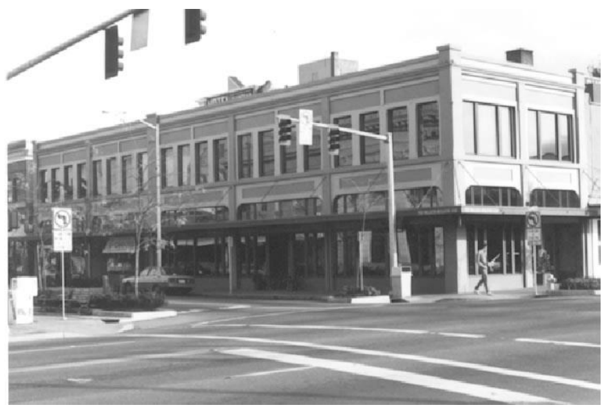
View of NW corner taken 10/16/1985 Photography Neg. No. (Roll No./Frame No.): 26-23A Comments:
