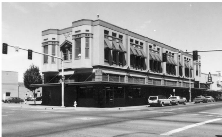
View of SW corner taken 7/1/1989 Photography Neg. No. (Roll No./Frame No.): 31-20 Comments:
