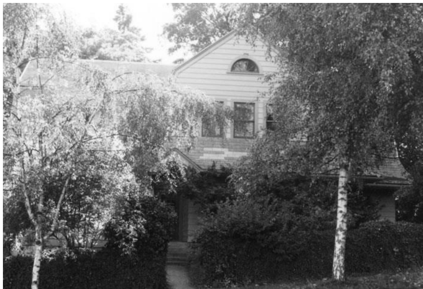
View of north facade taken 10/4/1985 Photography Neg. No. (Roll No./Frame No.): 23-28A Comments:
