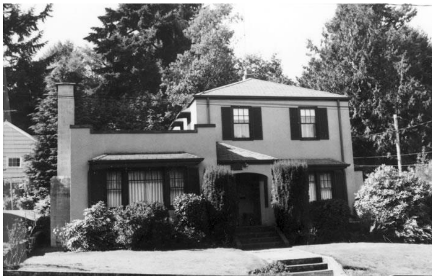
View of east facade taken 10/4/1985 Photography Neg. No. (Roll No./Frame No.): 23-27A Comments:
