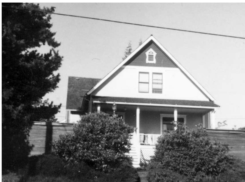
View of east facade taken 9/1/1997 Photography Neg. No. (Roll No./Frame No.): 43-27 Comments:
