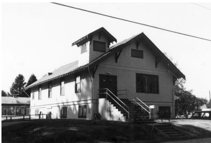
View of southeast corner taken 10/3/1985 Photography Neg. No. (Roll No./Frame No.): 23-1A Comments:
