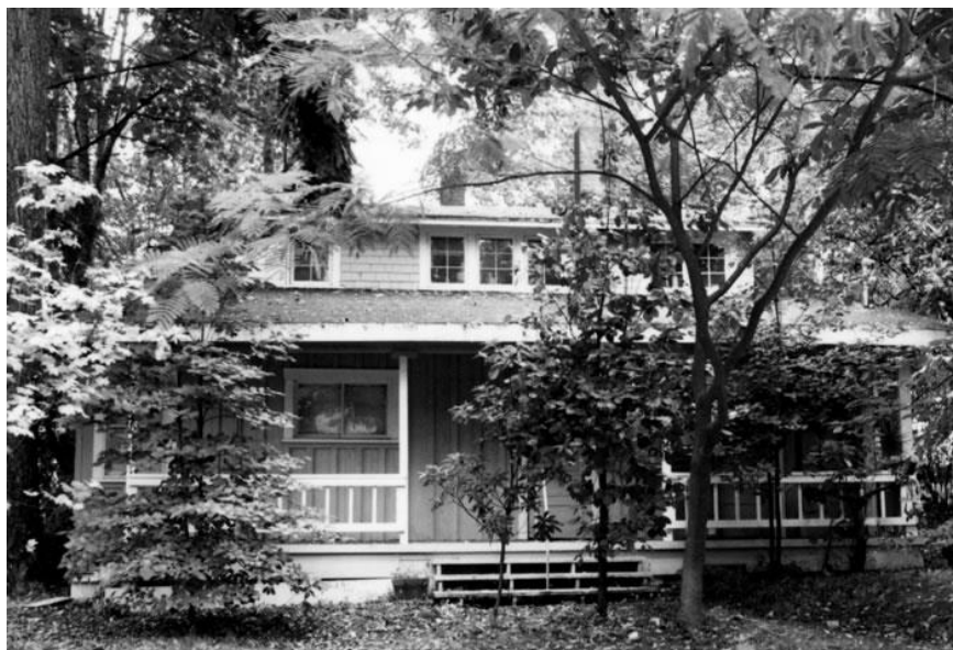
View of east facade taken 10/2/1985 Photography Neg. No. (Roll No./Frame No.): 22-8A Comments:
