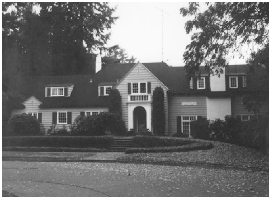
View of north facade taken 9/27/1985 Photography Neg. No. (Roll No./Frame No.): 21-34A Comments:
