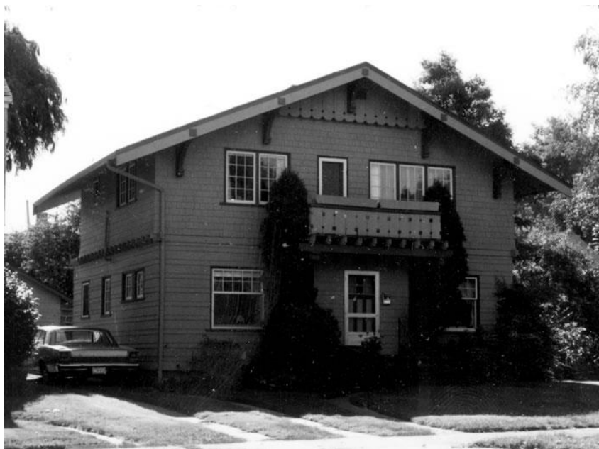
View of NE corner taken 9/26/1985 Photography Neg. No. (Roll No./Frame No.): 20-14A Comments:
