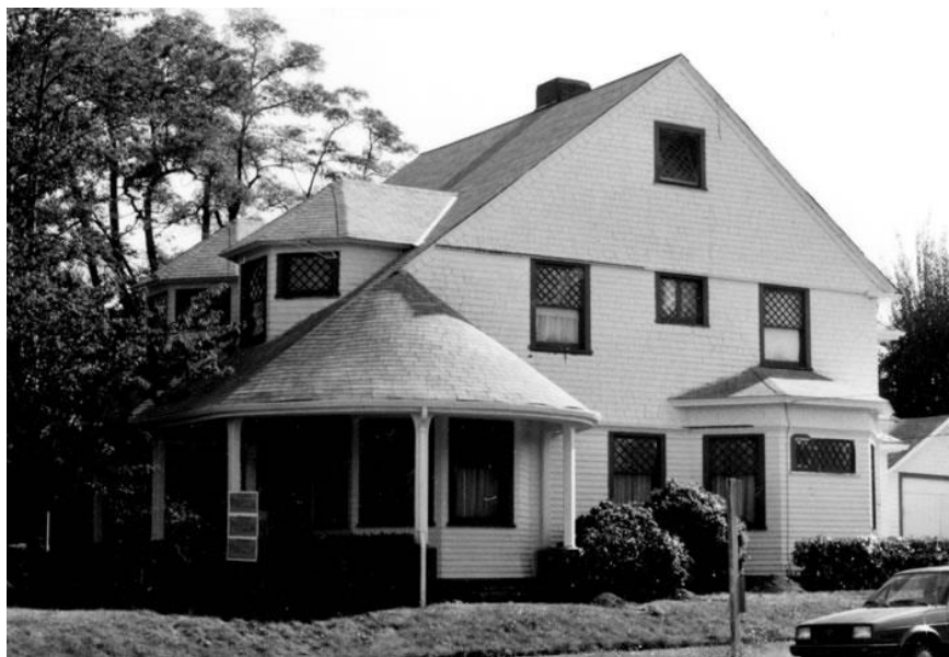
View of NW corner (shown), SW corner taken 9/26/1985 Photography Neg. No. (Roll No./Frame No.): 20-10A. 11A Comments:
