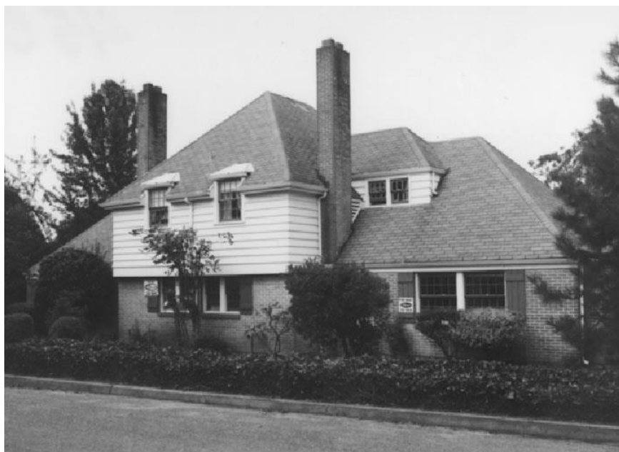
View of south facade taken 9/20/1985 Photography Neg. No. (Roll No./Frame No.): 19-3A Comments:
