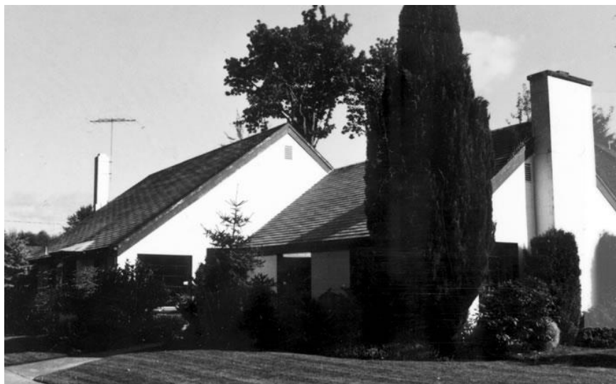
View of NW corner taken 9/18/1985 Photography Neg. No. (Roll No./Frame No.): 18-6A Comments:
