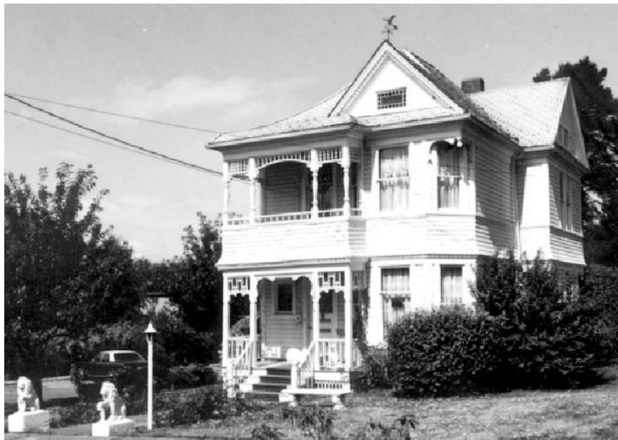
View of SE corner taken 9/11/1985 Photography Neg. No. (Roll No./Frame No.): 16-12A Comments:
