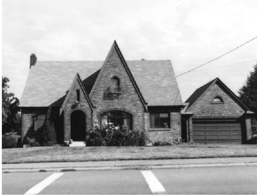
View of south facade taken 9/11/1985 Photography Neg. No. (Roll No./Frame No.): 16-2A Comments:
