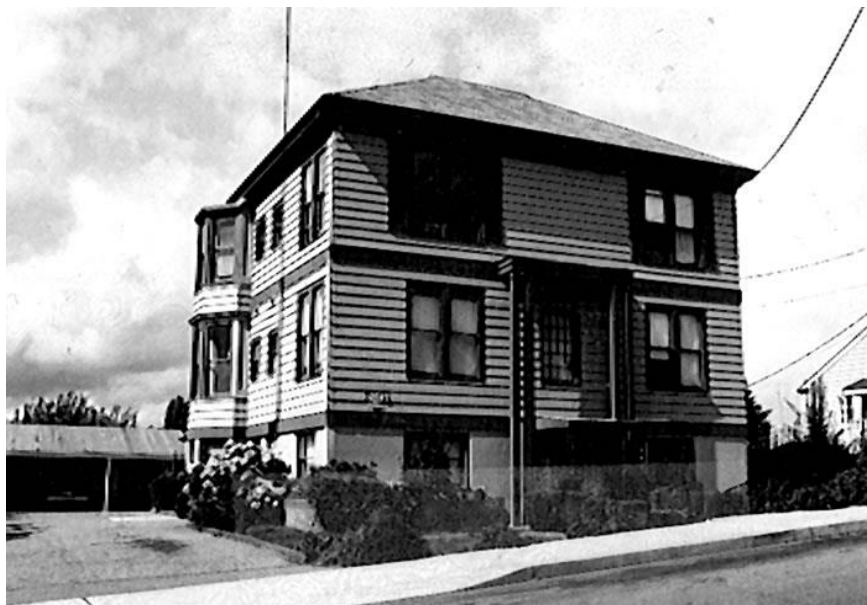
View of East facade taken Photography Neg. No. (Roll No./Frame No.): 45-28 Comments:
